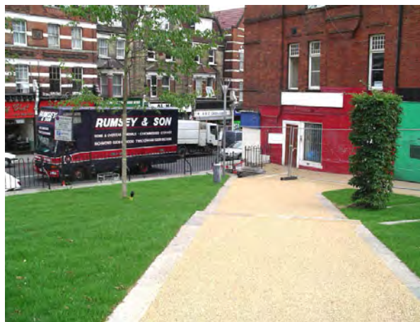
Resin-bonded gravel used at Streatham Green
