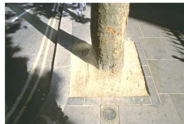
Tree detail using bound gravel and discreetly detailed irrigation tube/aeration tube
