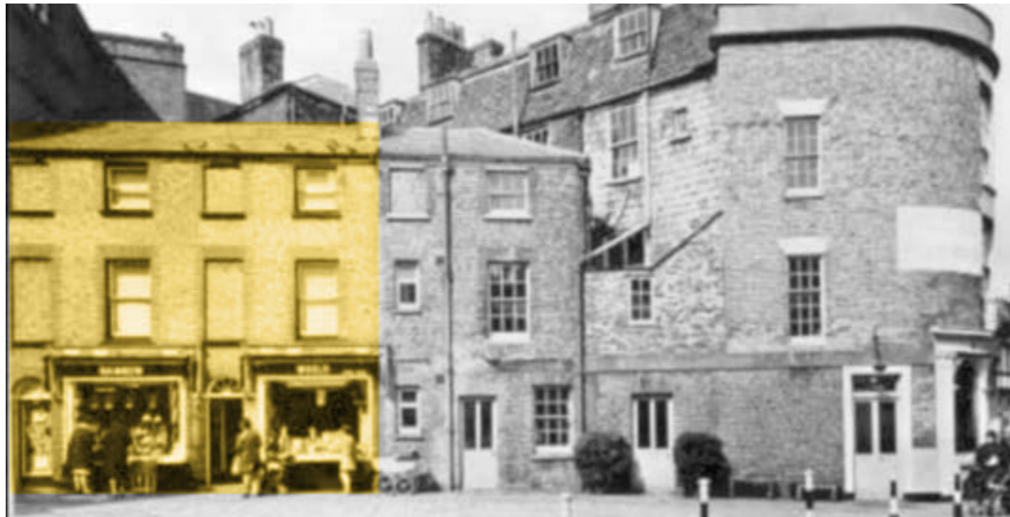
Historical image showing the relationship between the shop fronts of nos. 25-26 St Thomas's Square (highlighted) and the original Eagle Tavern building
