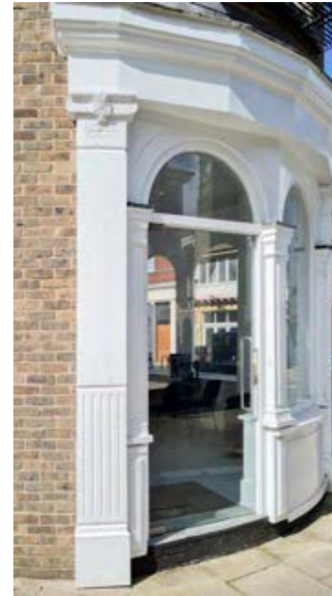
The principle of using decorative pilasters and consoles (left) to demarcate individual shop fronts has been retained using replacement fixtures that complement the detailing of the former public house (right) along the High Street frontage
