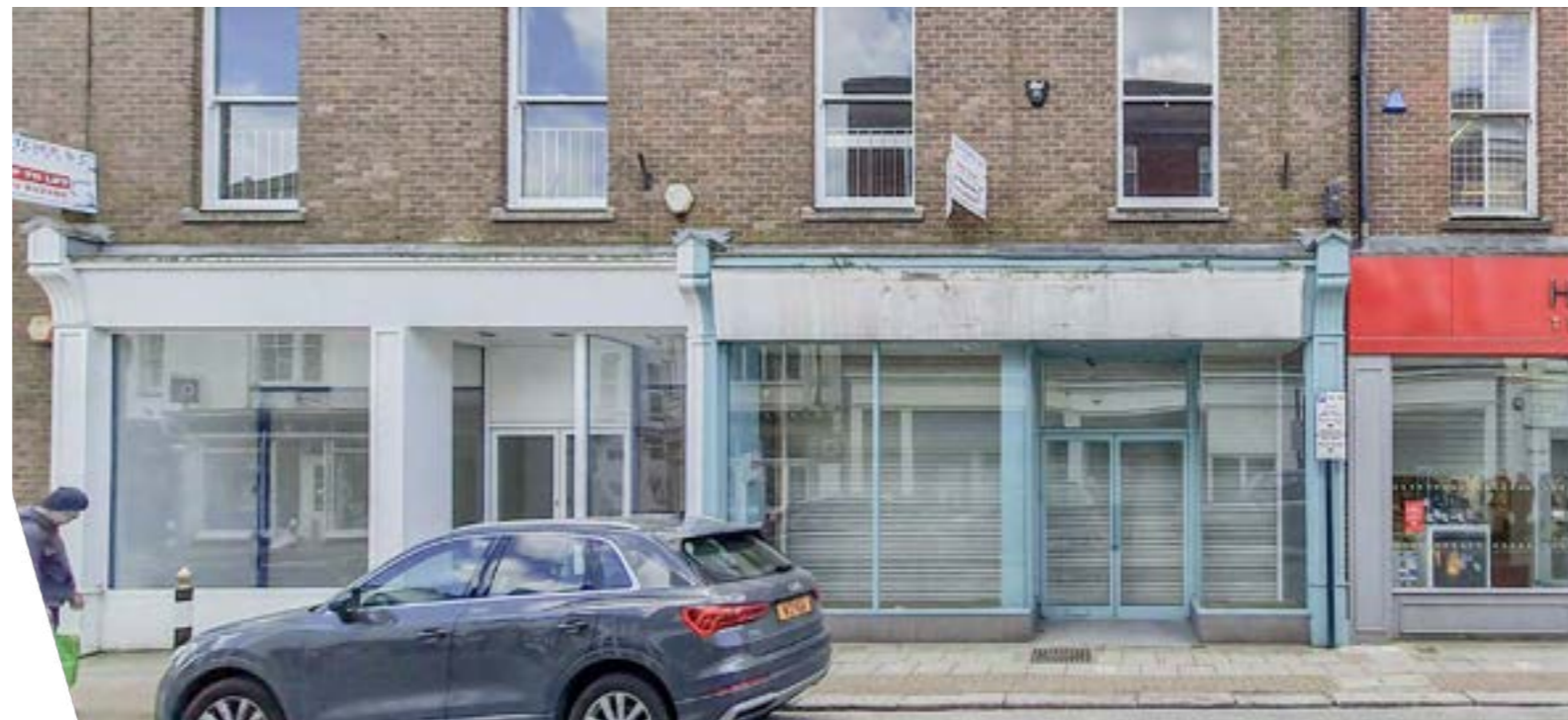
Decorative pilasters reinforcing the Victorian parade style rhythm of the original shop fronts
