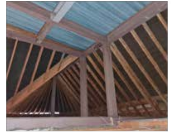
The existing mansard (modern) roof structure above units 35 and 36 is comprises a composite of ribbed steel sheets attached to timber plates atop I section beams with sufficient head room
