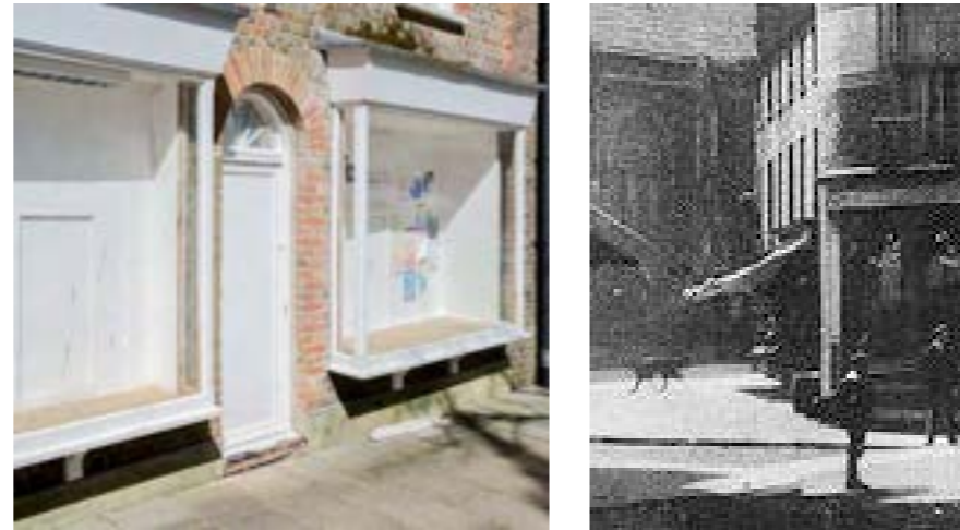
Replicated Georgian square bay windows to 25-26 St Thomas's Square (above left) with historic shop frontage shown below and with blinds extended (above right)
