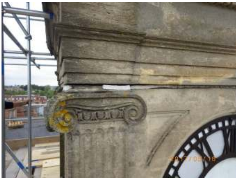
Figure 4: Detail of clock tower 2017
