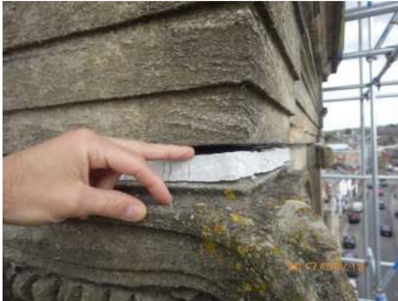
Figure 5: Detail of clock tower 2017
