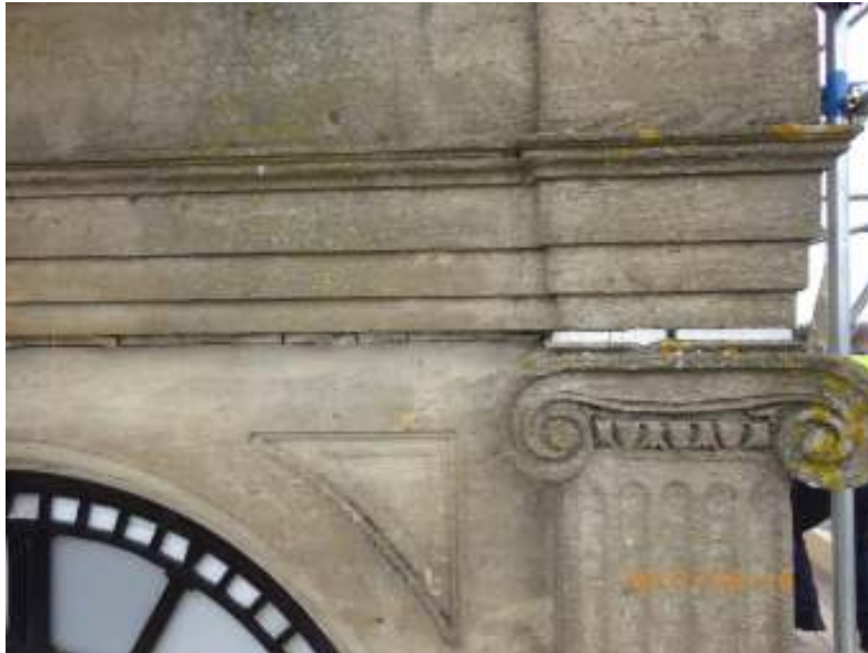
Figure 3: Detail of clock tower 2017
