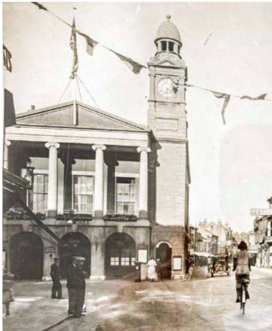
1935 photograph showing public toilets installed at ground floor alongside fire and ambulance stations
