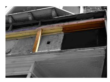
An example of an additional horizontal, timber batten supported by vertical post and used to achieve an angled fascia.
