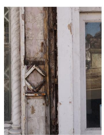
The effects of poor maintenance can clearly be seen on this shopfront joinery
