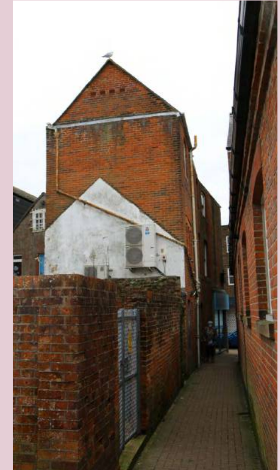
Above, right: the southern end of Post Office Lane, looking towards High Street, the electricity sub station is to the left.
