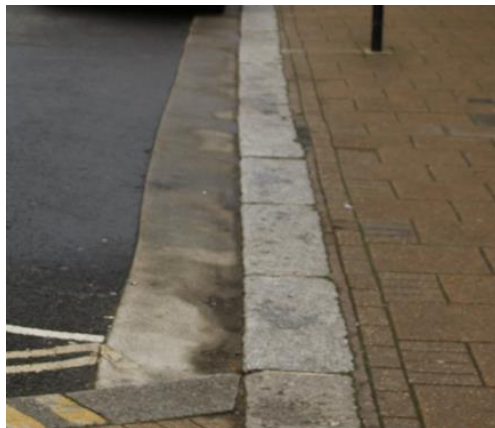
Figure 7.7. Kerb style, in order of priority, left to right: 1) retain existing granite kerbs and channel blocks, 2) new additional granite kerbs were necessary, 3) Conservation kerbs in lower priority areas subject to cost.
