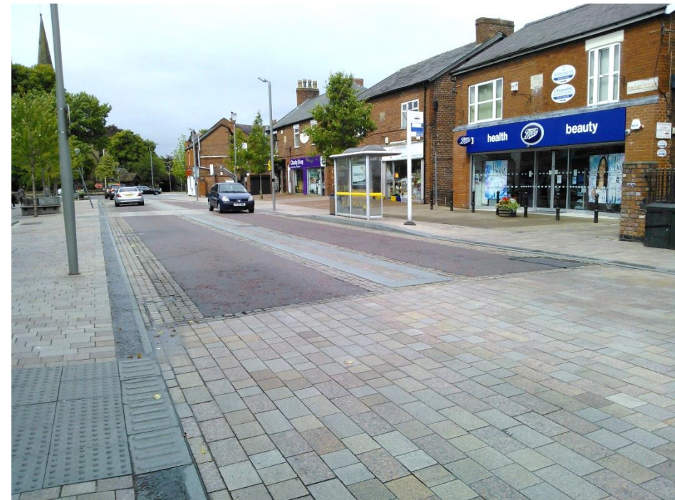
Figure 5.3.: Informal crossing point over Park Lane, the main High Street in Poynton, Cheshire, with the same streetscape treatments used on connecting A Roads.
