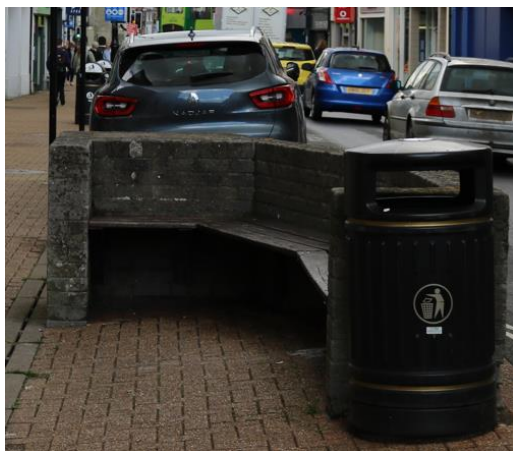
Existing brick-built seating to be replaced.
