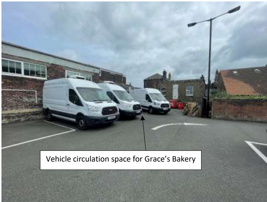
Figure 8.1. Photograph of Victoria Street Car Park, looking towards Grace's Bakery Parking bays and narrow lane to back of 176 and 177 High Street, taken May 2022.
