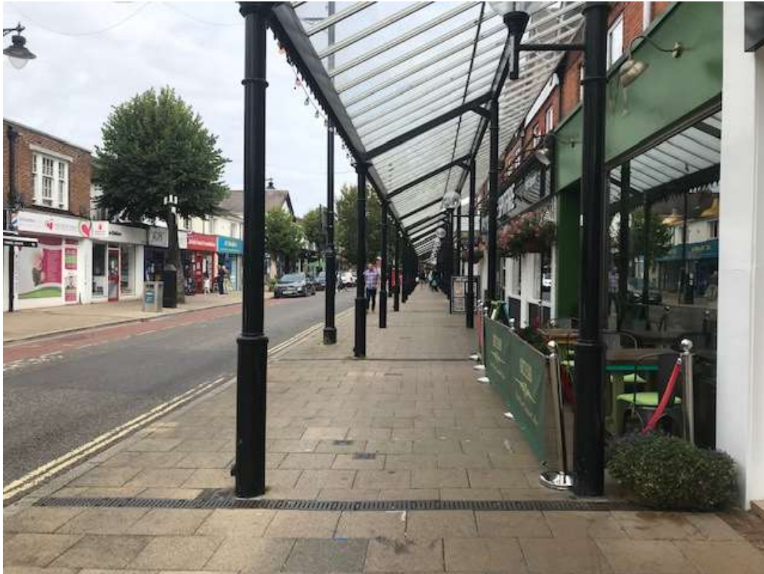
Figure 5.6. Arcades adjacent to the pedestrian area. Note: arcade support posts are for the most part situated at regular intervals of around 4ms and are clear of the drainage channels.
