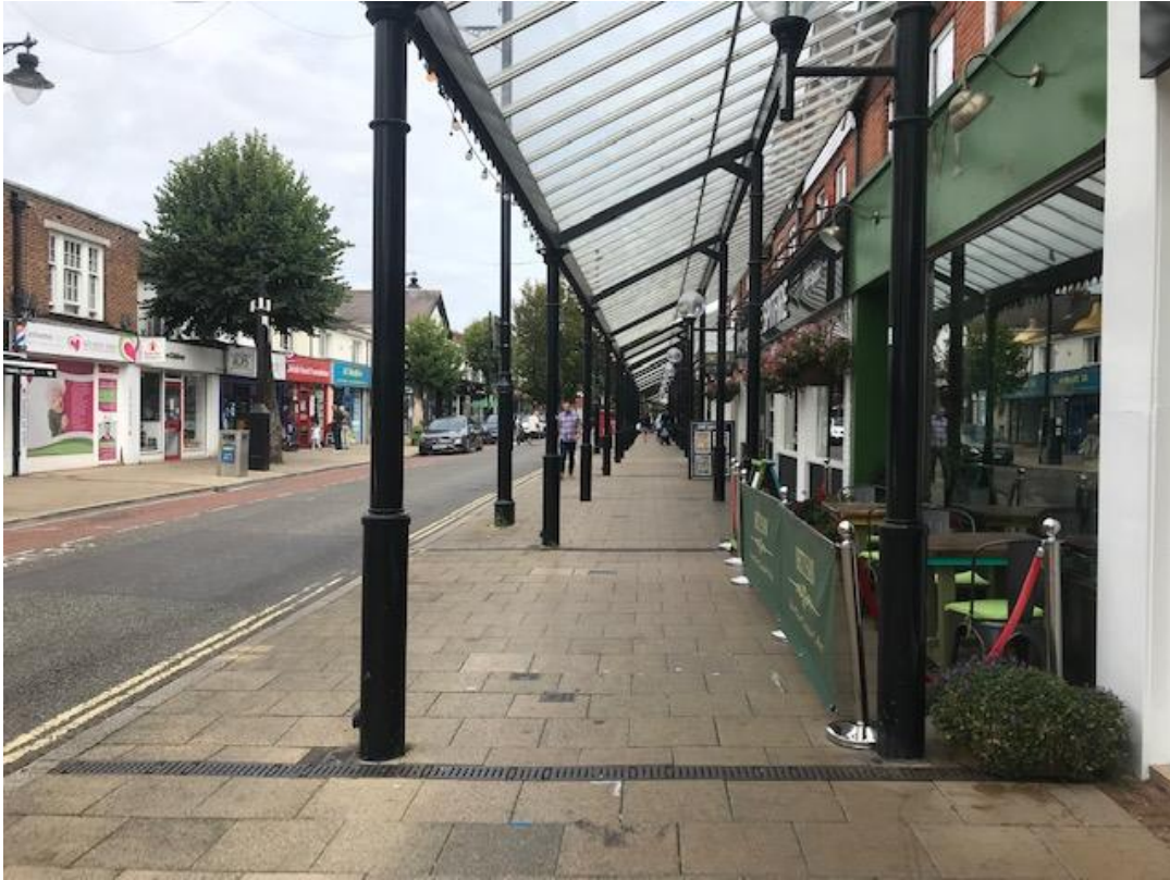
Retrofit free standing arcades in Eastleigh, Hampshire
