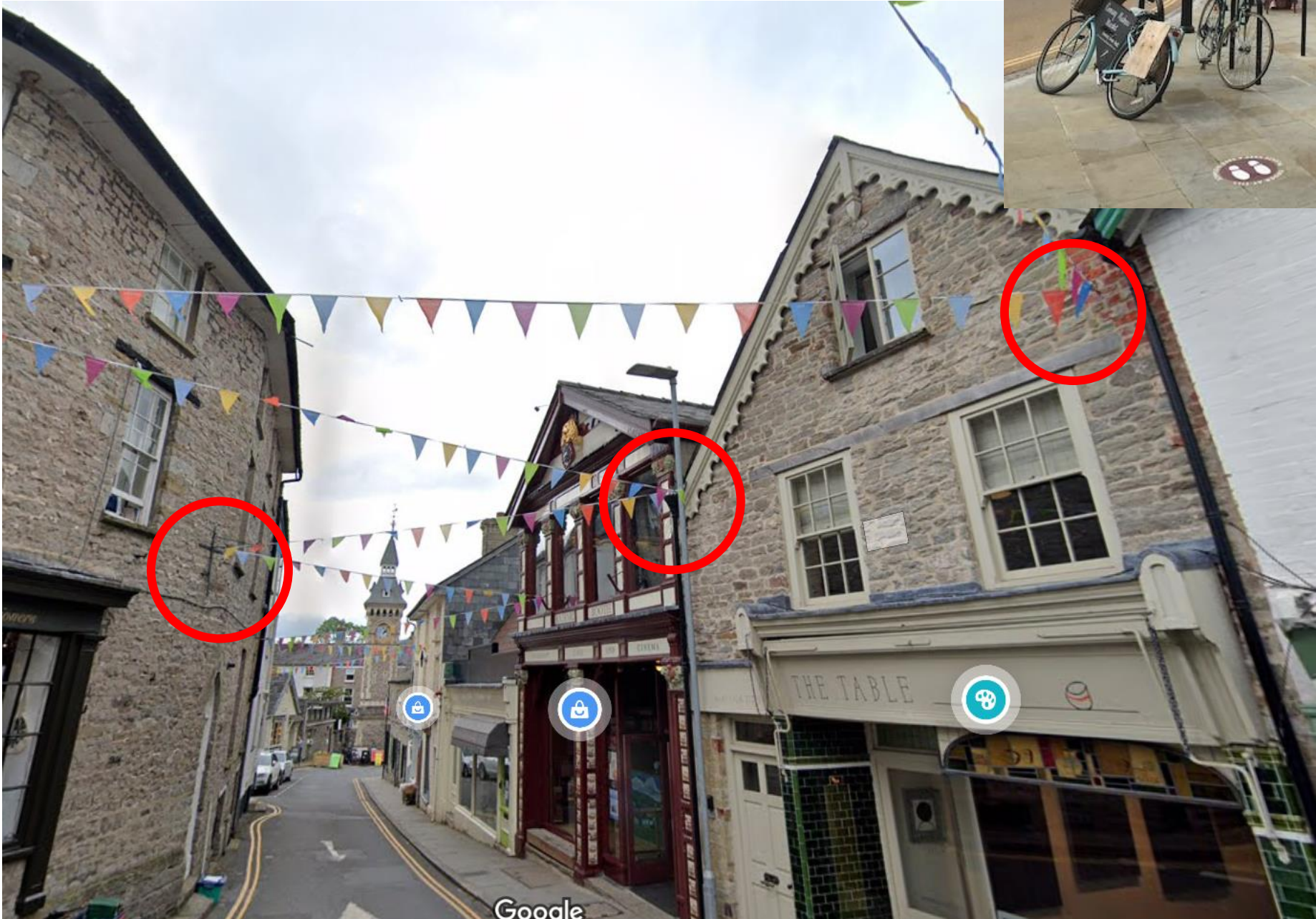
Bunting in Hay-on-Wye (image from Google Streetview): note varied attachment details not recommended.
