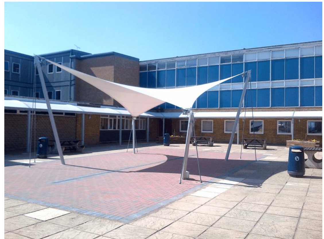
Example of sail structure held in place by tensioned cables and steel poles
