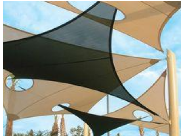
Sail Awnings, attached by tensioned cables to steel poles
