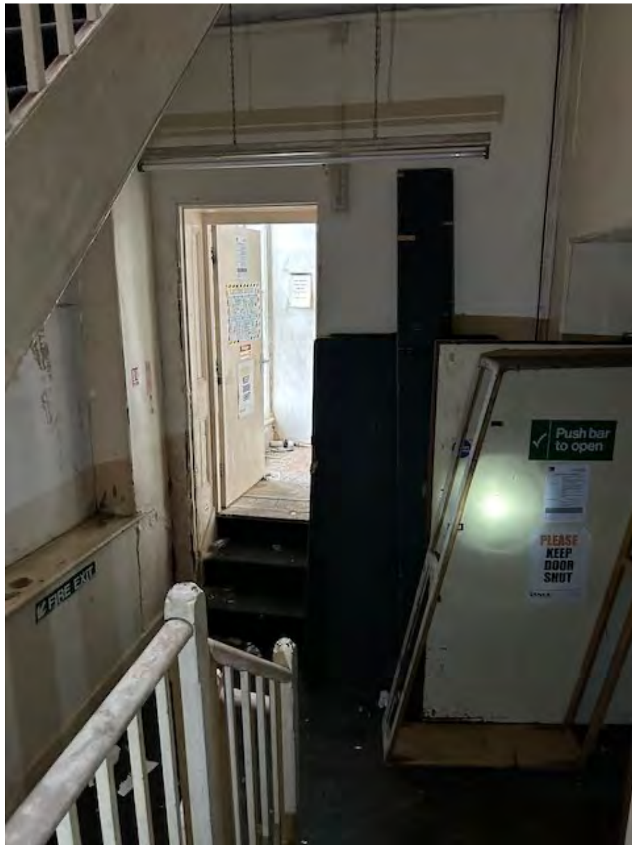
East service staircase C19.
