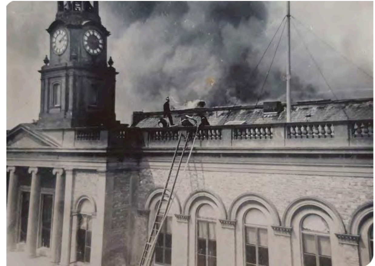
June 1931: Fire destroys the roof, and substantial damage to the building
