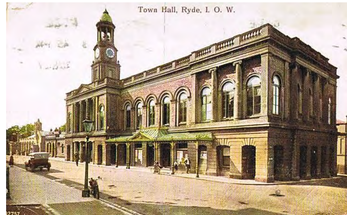
Figure 1 South Elevation Circa Early 20th Century Showing the Glass Canopy Removed in 1950
