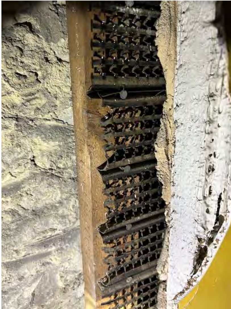
1930's dry lining with Plaster of Paris pilaster strips
