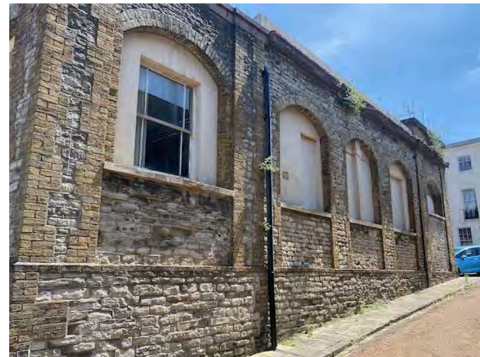
West elevation windows
