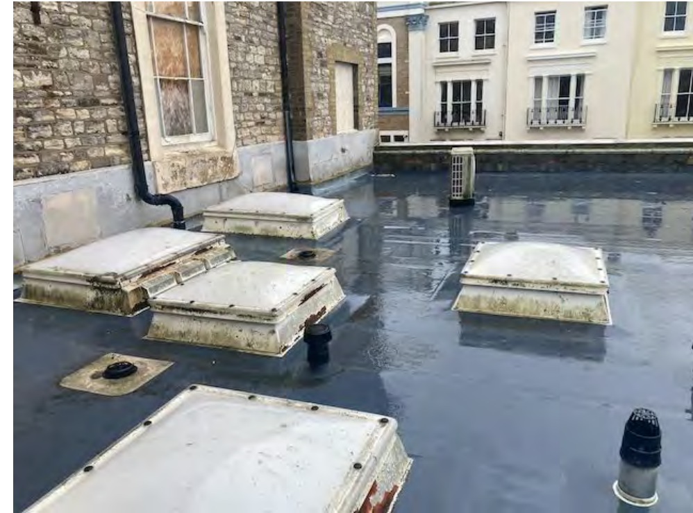
Flat roof over the western office accommodation
