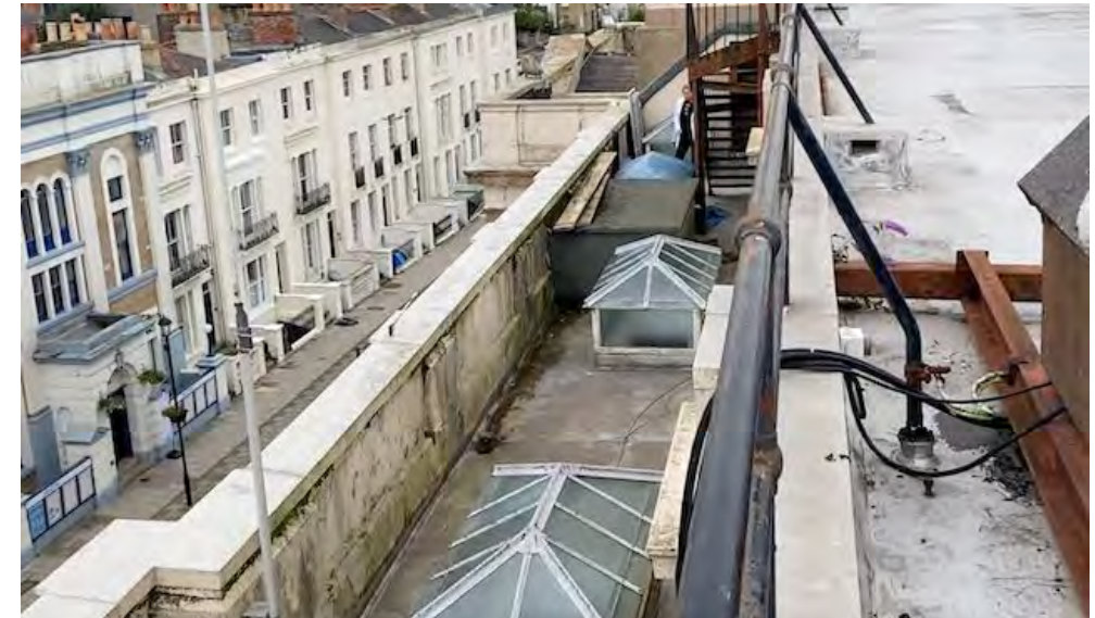
Smaller flat roof with five lanterns and the cast iron stairs
