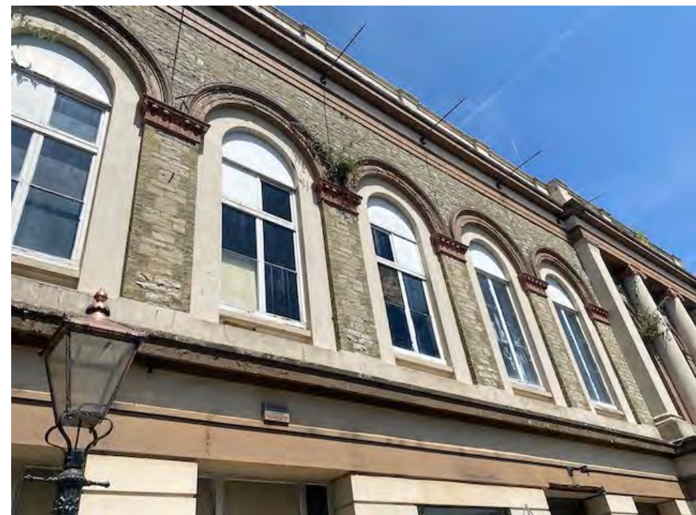
The first floor windows showing moulded acanthus leaf capitals
