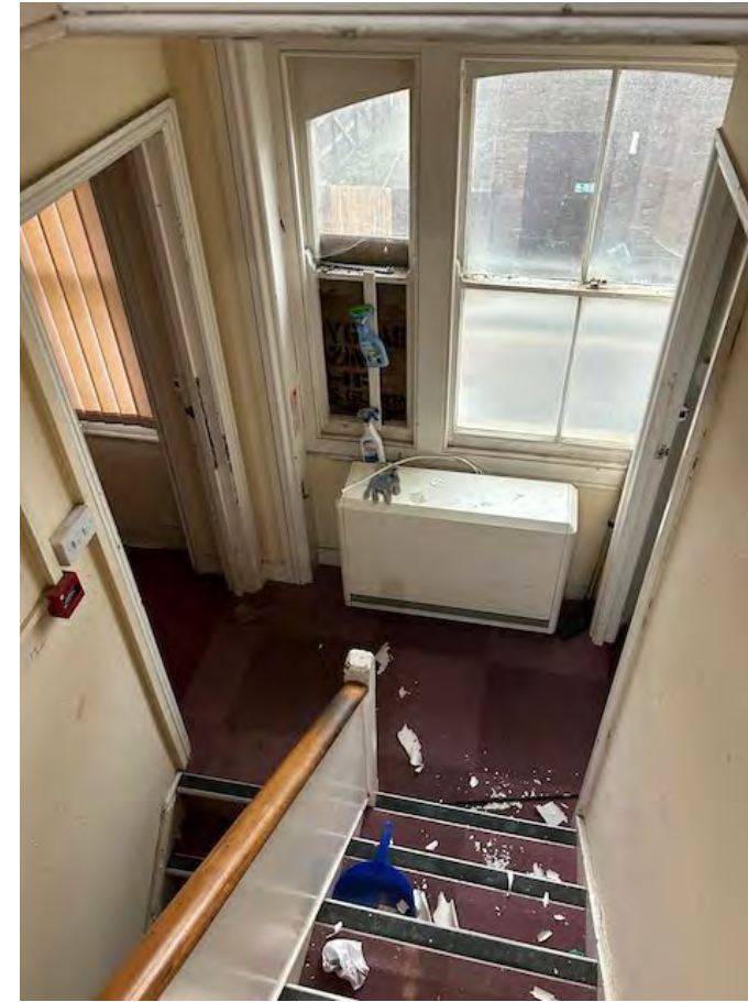
Central staircase leading to caretakers accommodation
