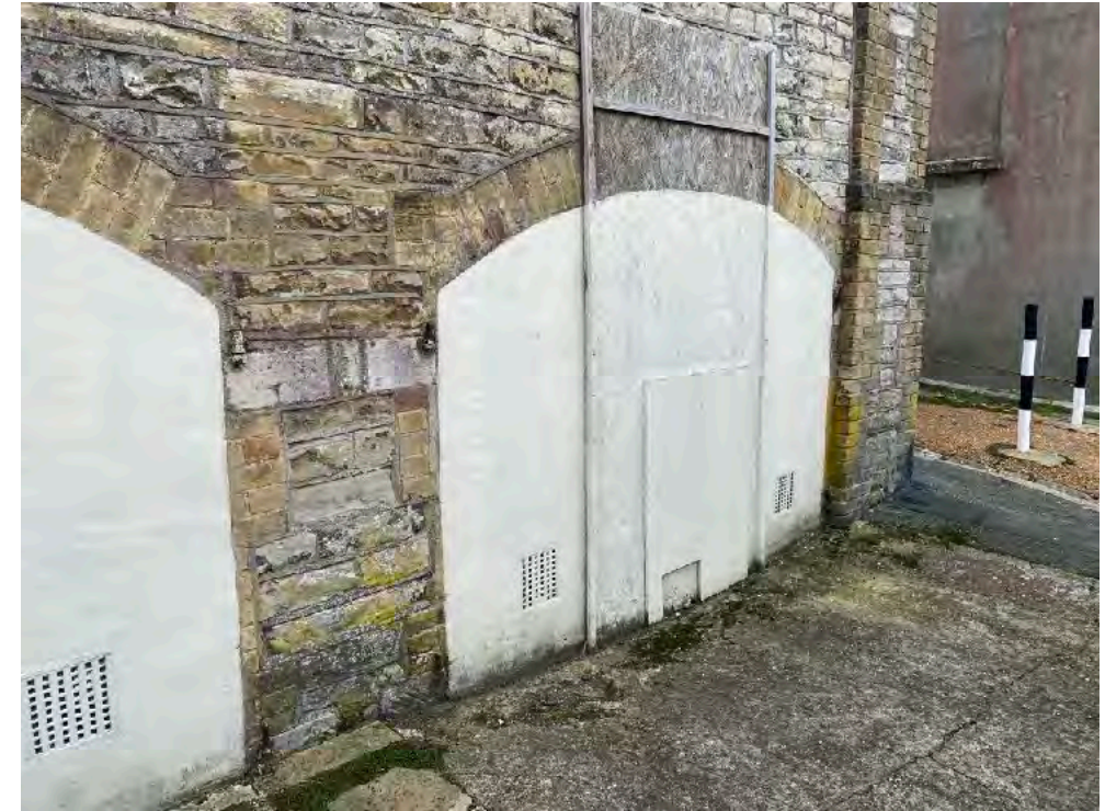
Rendered panels that may have previously contained doors to an undercroft.
