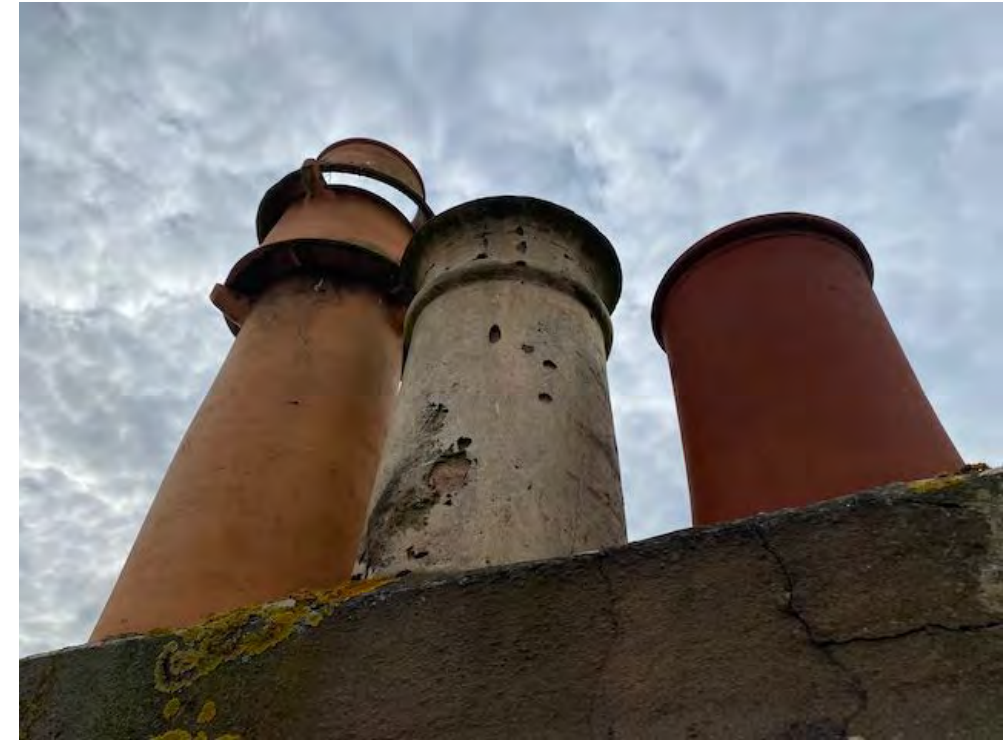
Chimneys serving the flat
