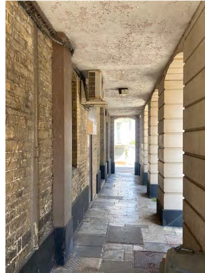
Inner wall of the eastern arcade
