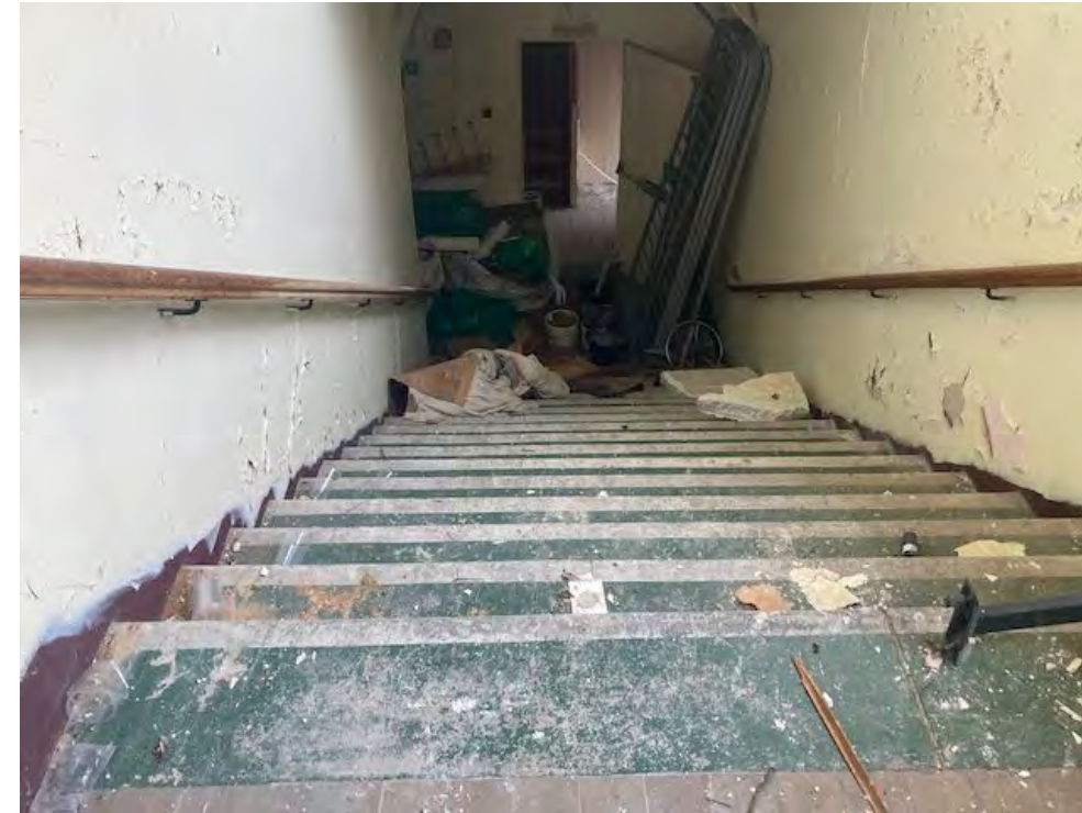
Stairs leading from lobby to street exit
