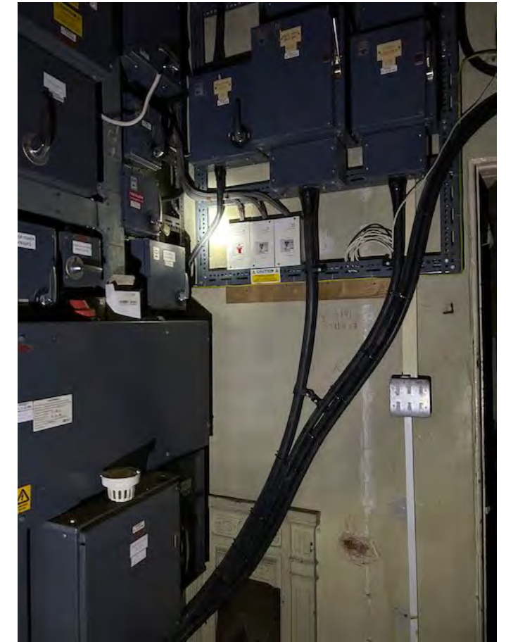
Note historic fire surround below
