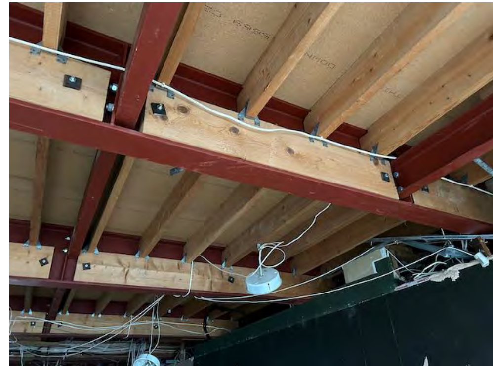
The steel frame of the mezzanine
