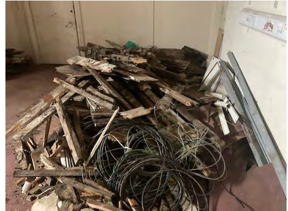
Removed dry rot damaged flooring stored on ground floor risking further contamination.
