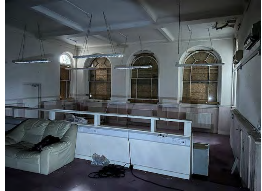
Lower main hall looking north
