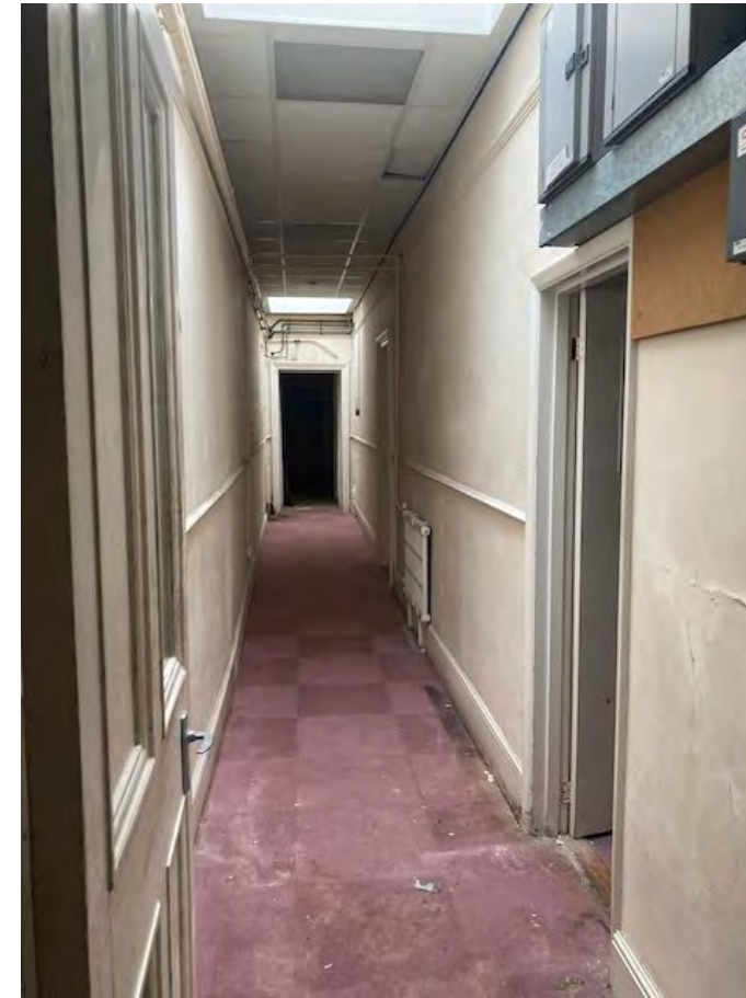
Corridor in western single storey accommodation. Modern suspended ceiling
