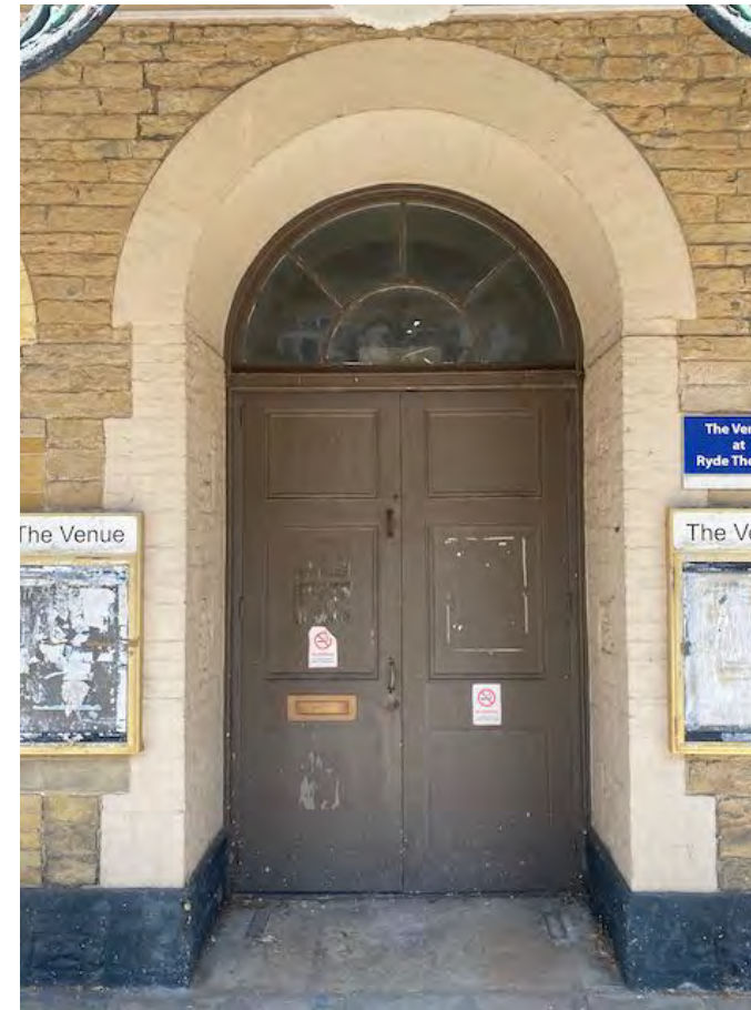
Main entrance doors
