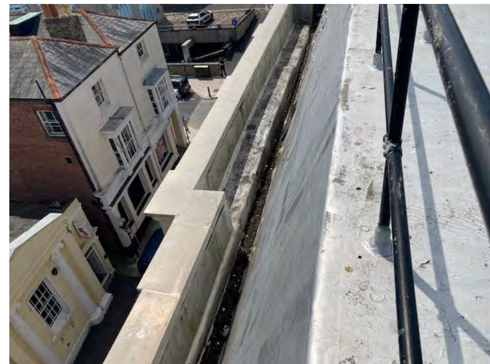
The Mansard Roof
