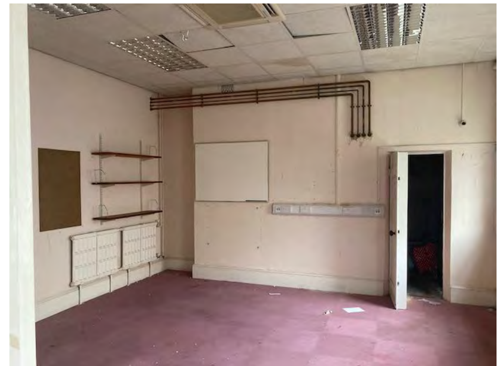
G18: Strong room door to East wall.
