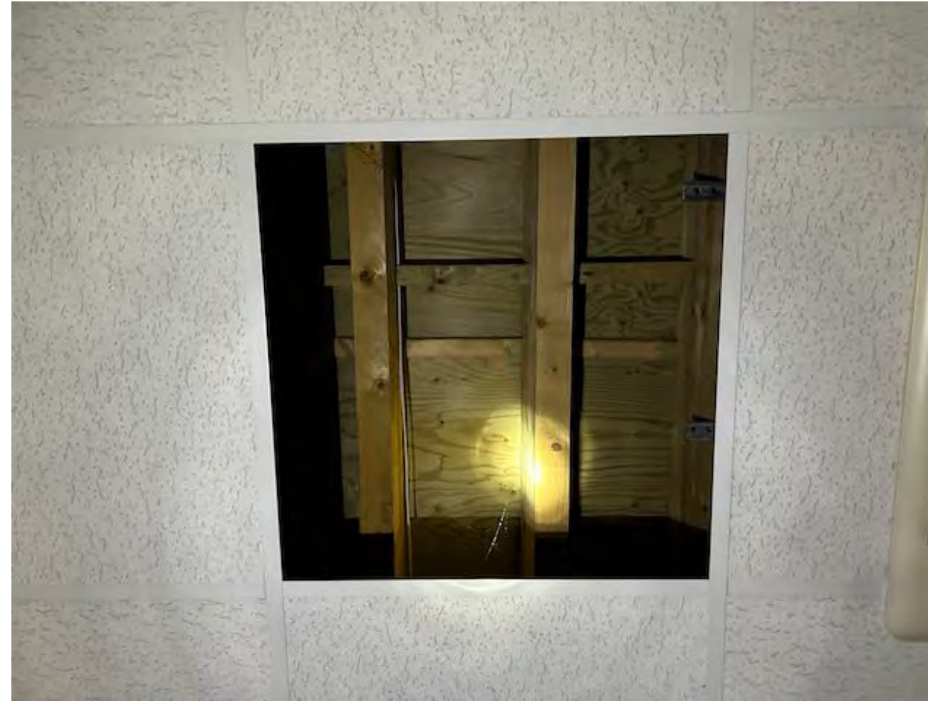
Modern roof construction beneath the West Range offices
