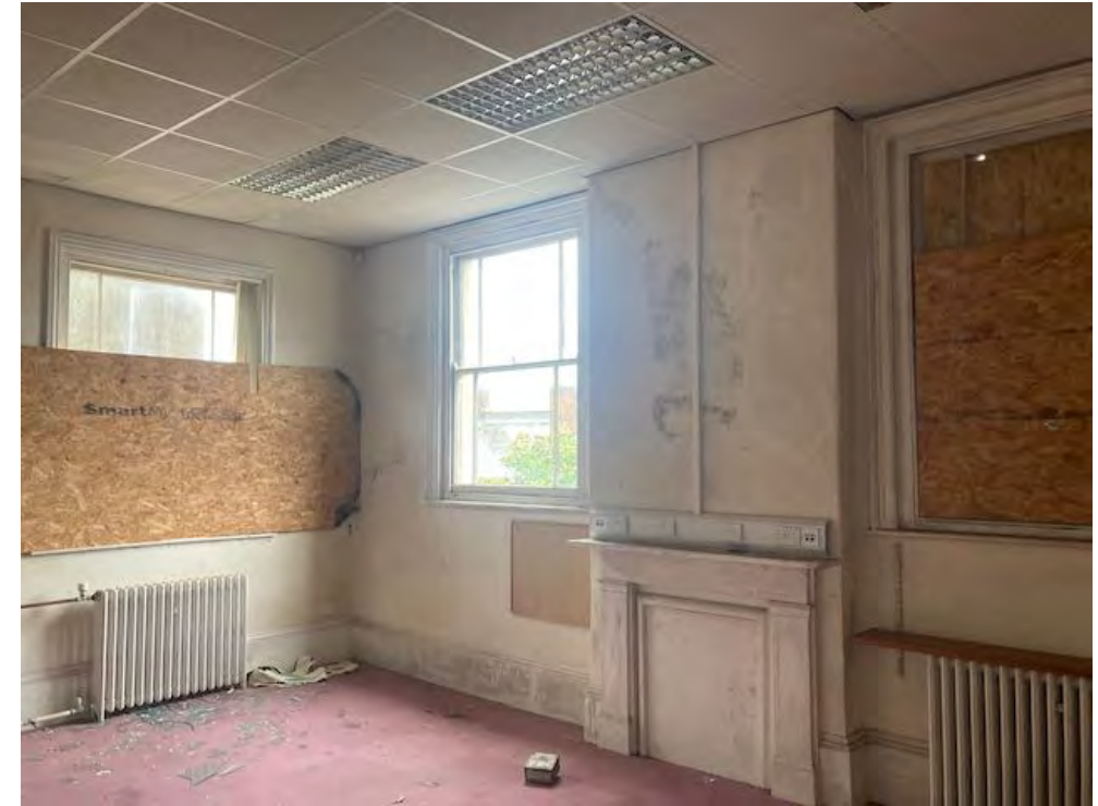
Sash windows on the north western corner
