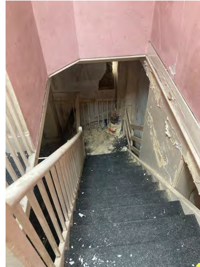
Performers' stairwell in south eastern corner
