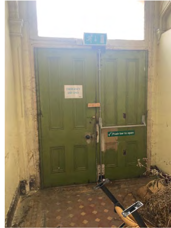
Ground floor entrance from Green Stair Exit to Lind Street
