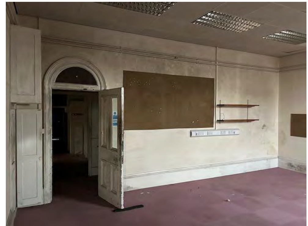
Office in the north west corner of the building
