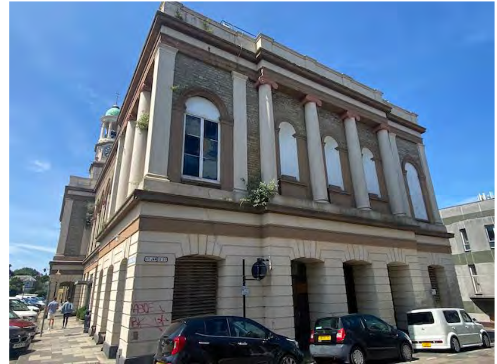
Eastern elevation showing the partially open arcade at ground level
