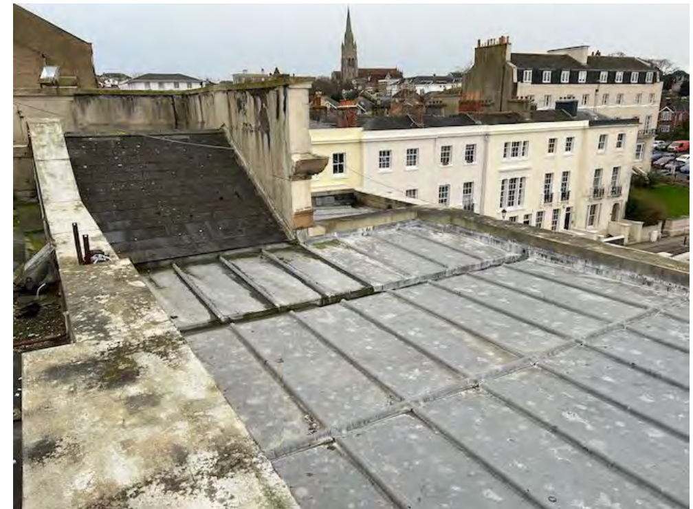
Lead roof above the Council Chamber
