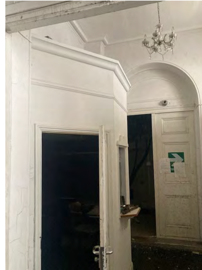
Central ground floor lobby area
