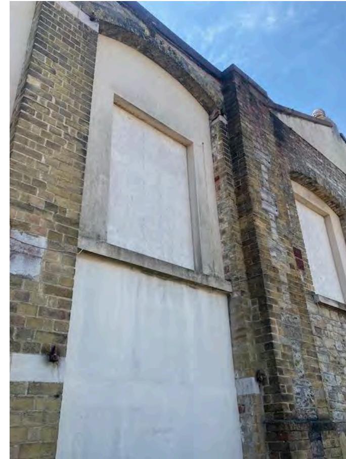
Closed openings with iron pintels
