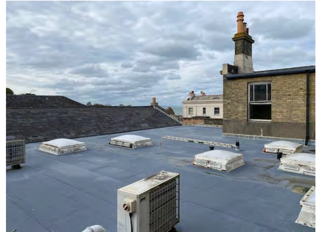
Flat roof area over western office accommodation. Flat to north.
