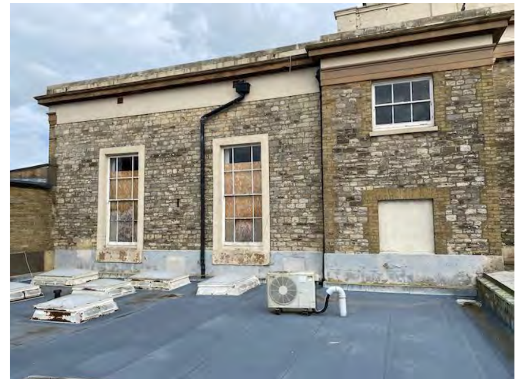
Walls of the west facing elevation of the Council Chamber
