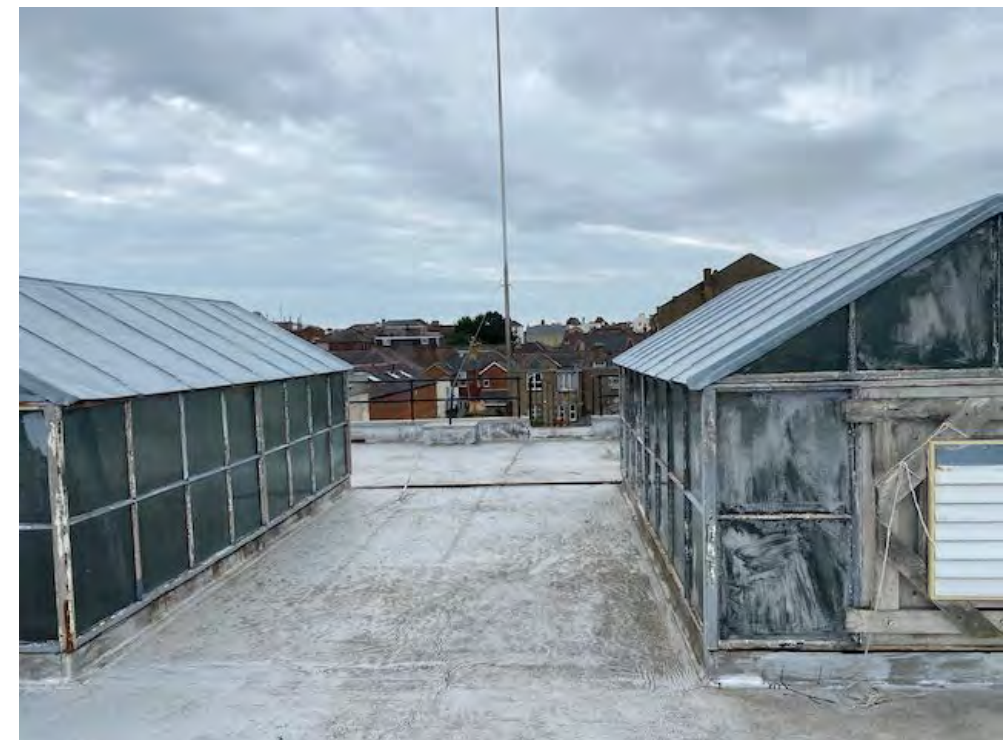
Main roof showing Georgian wired glass lanterns
