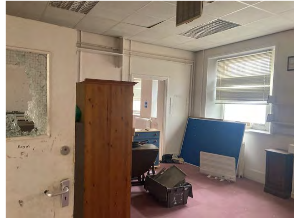
Office to west in the south elevation of the west wing
