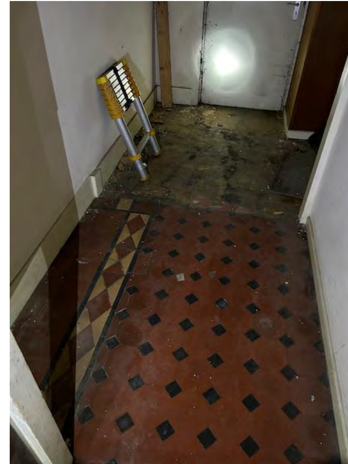
Entrance hall with the decorative tile finish
