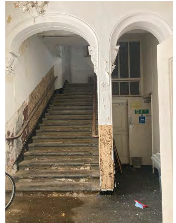
Main staircase to First floor
