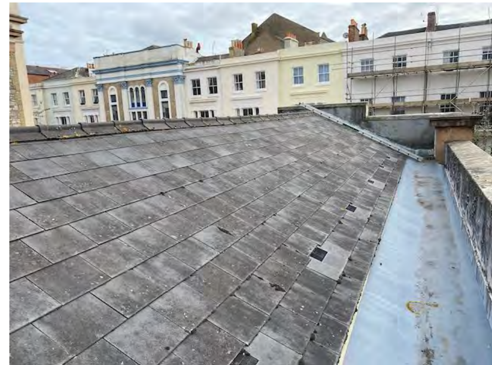
Pitched roof immediately west of the flat roof area
