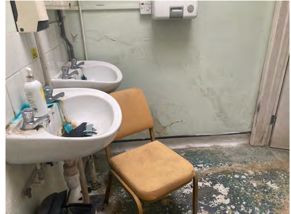
Lavatories in the eastern end of the west wing
