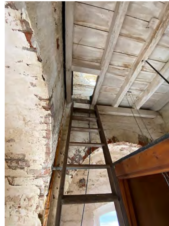
Wooden ladder providing access to clock face level
