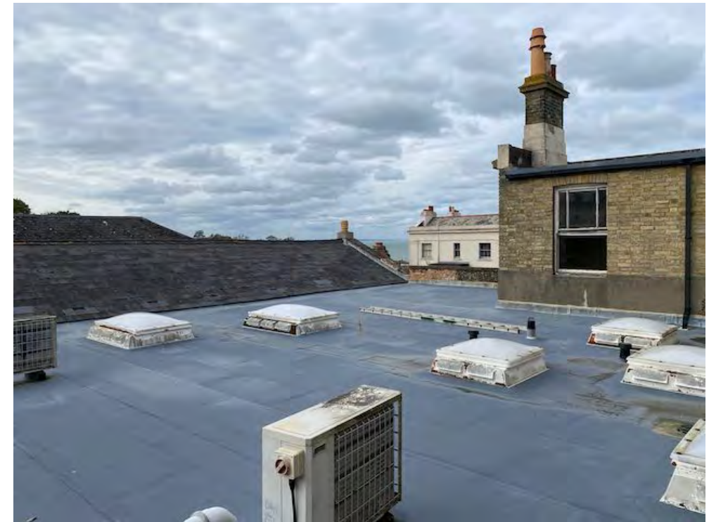
Flat roof between Council Chamber and the western pitched roof
