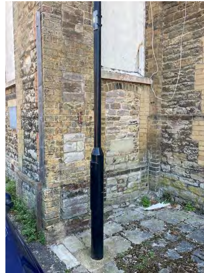
Blocked up former doorway
