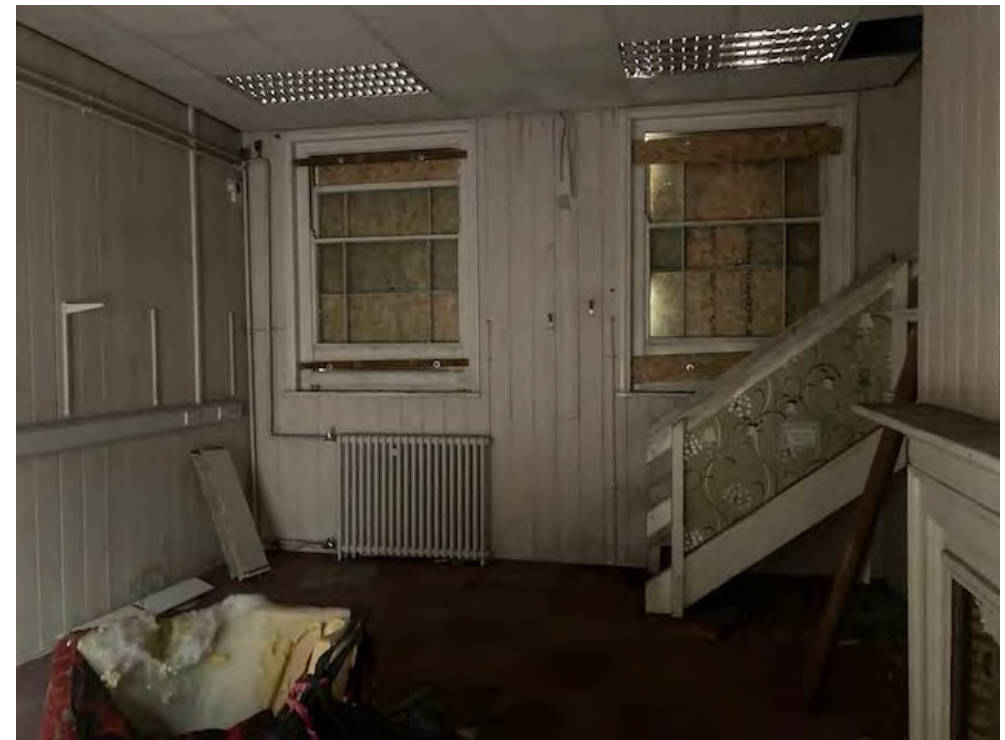
G10 office accommodation with suspended ceilings
