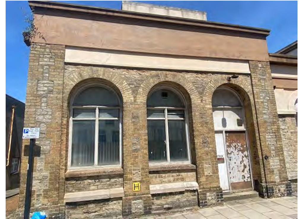
Windows at the eastern end of the southern elevation
