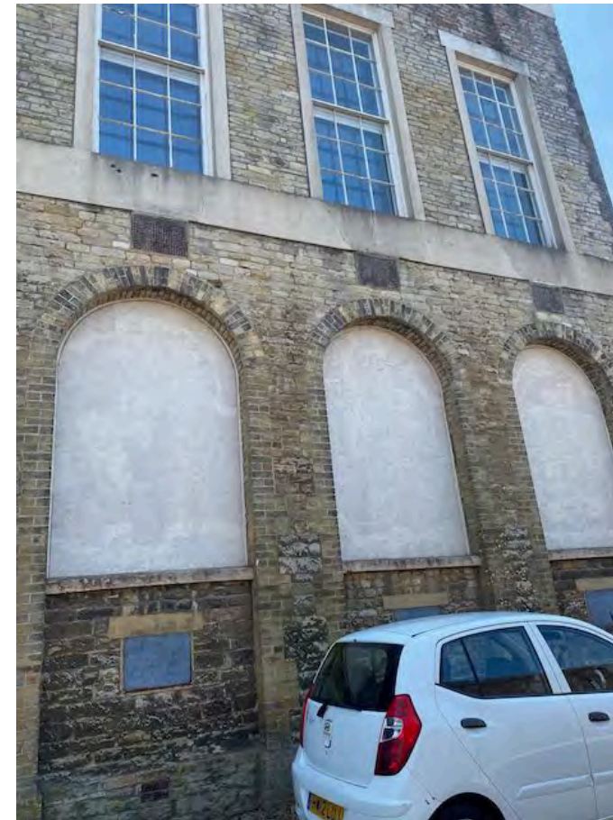
The projecting bay showing the three large openings
