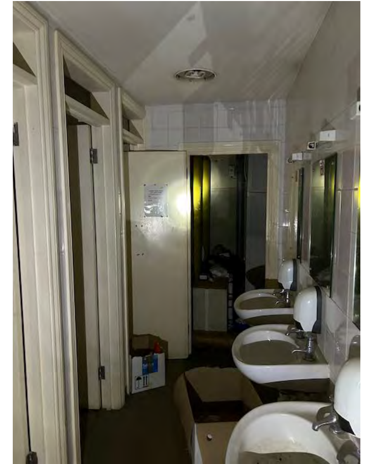
Toilets S9 with water cylinder cupboard beyond
