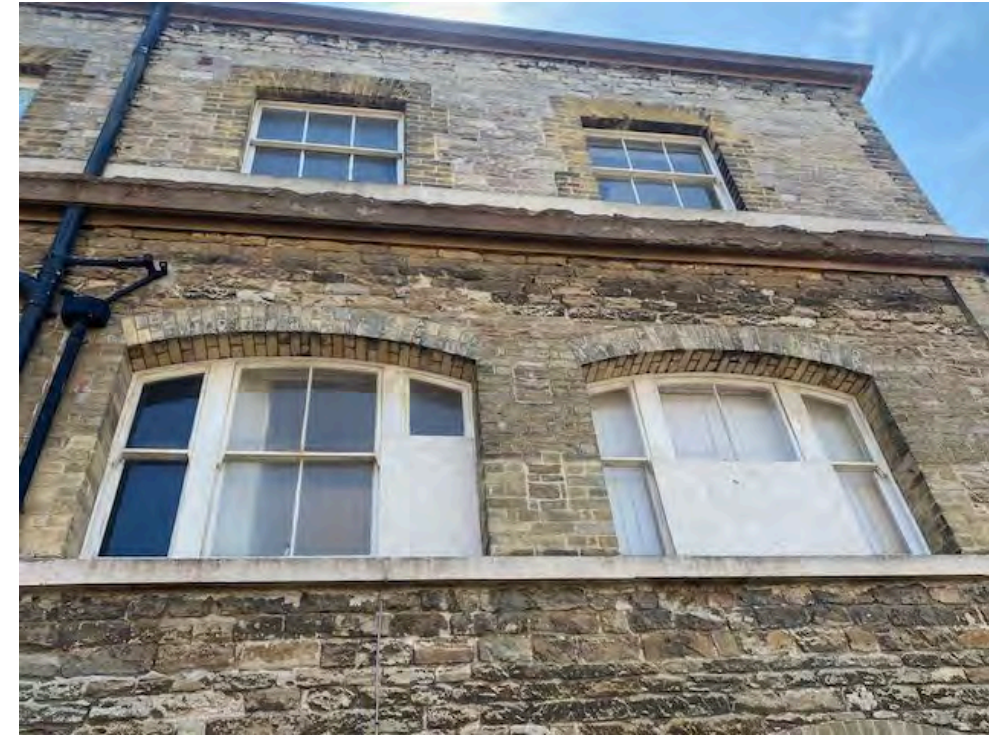
Windows on the market street elevation.
