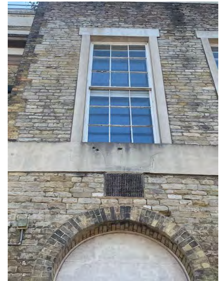
The rendered string course and one of the metal vents
