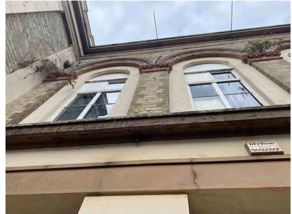
First floor windows with semicircular arched windows
