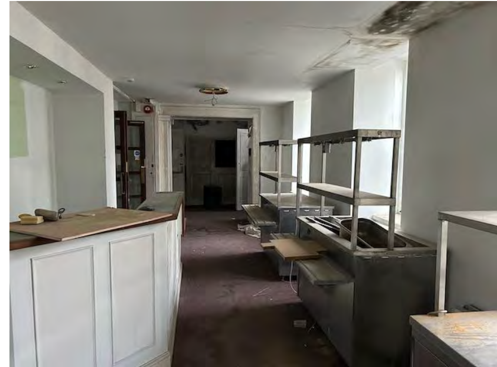
First Floor Foyer
