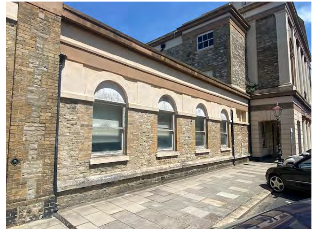
Windows on the link section
