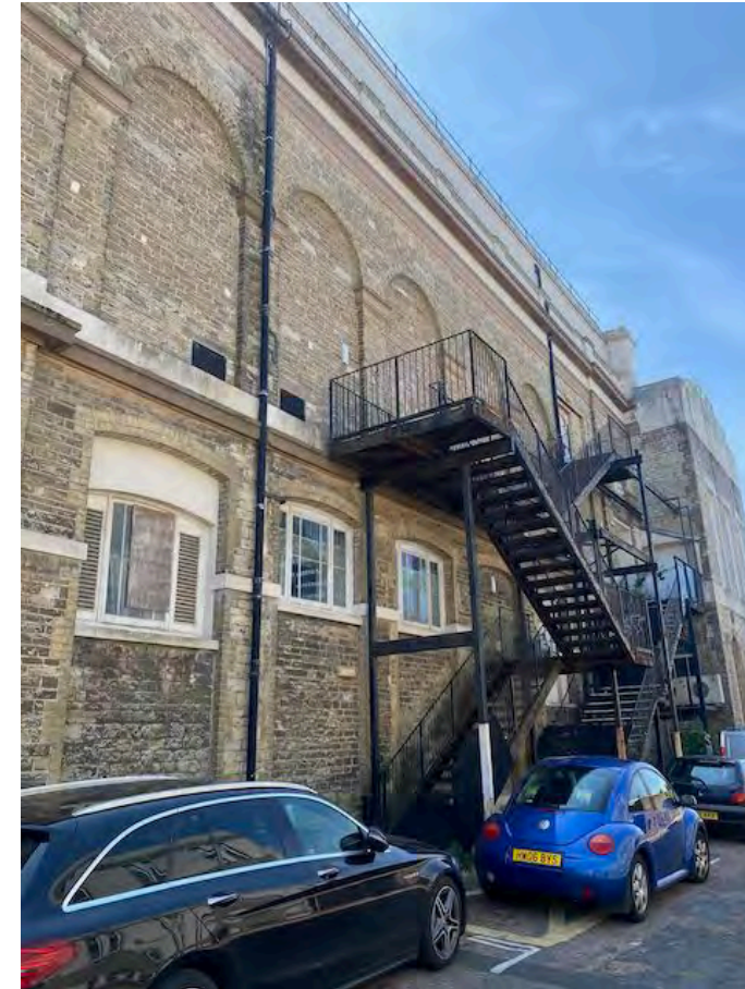
The north elevation
