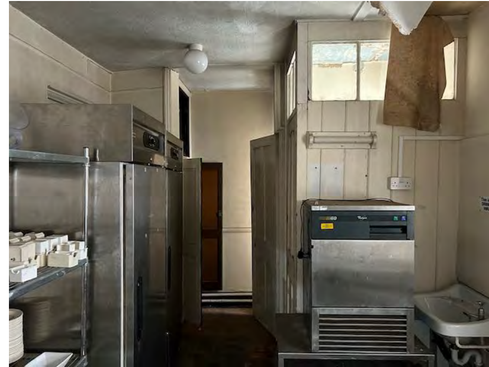
Ante Room looking west. Lavatories behind match boarding
