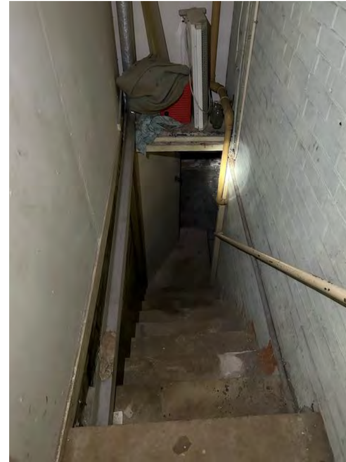
Access to boiler room
