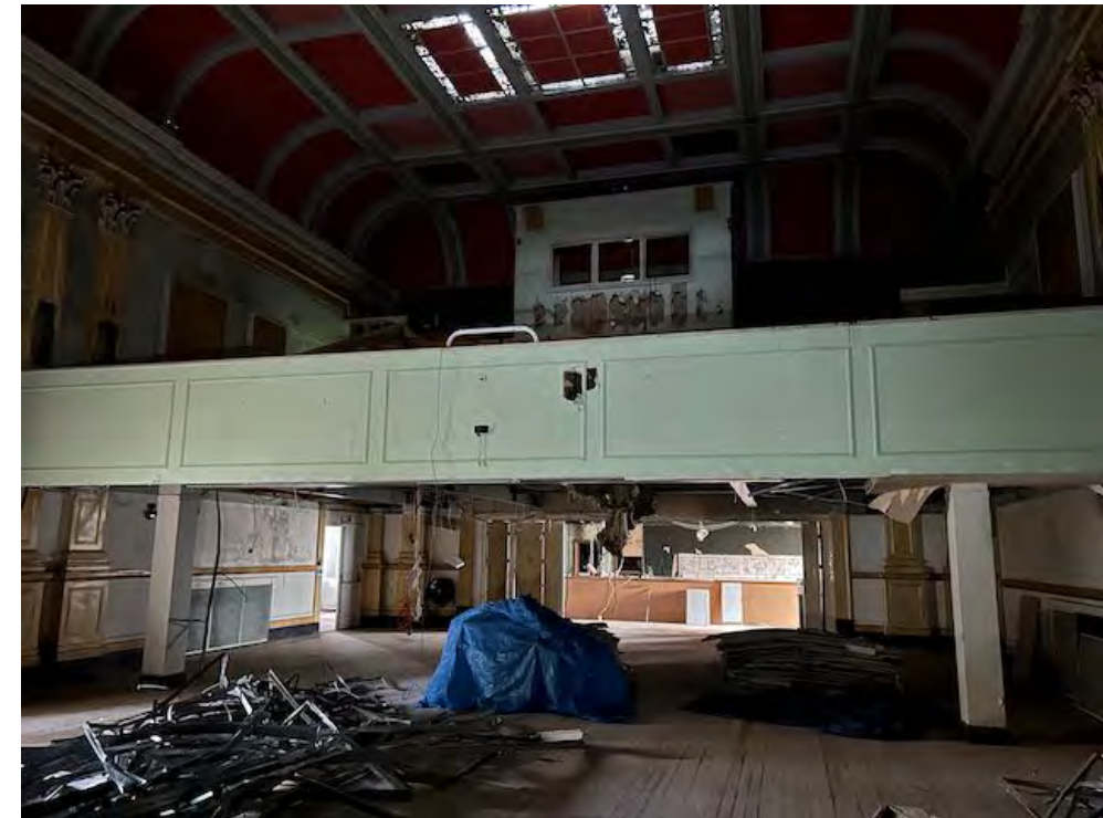
Auditorium and balcony
