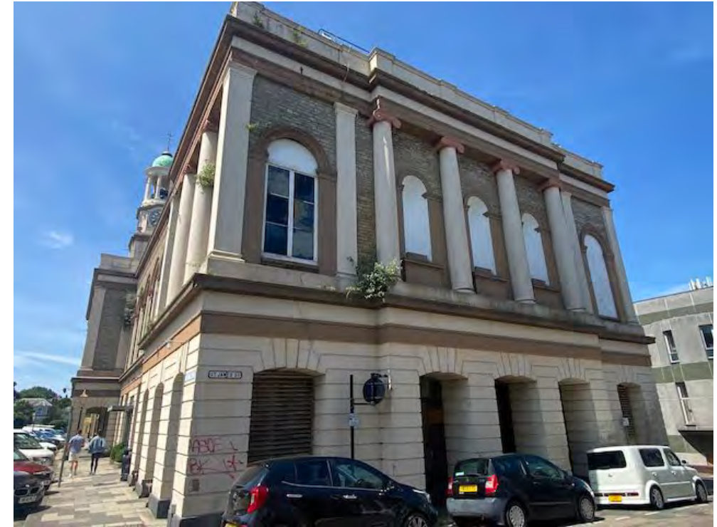
Ryde Town Hall from the East
