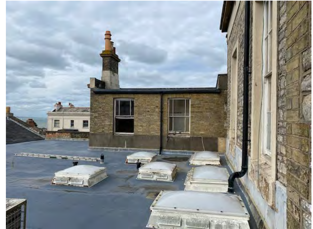
Flat roof generally in a good condition, with serviceable rooflights.
