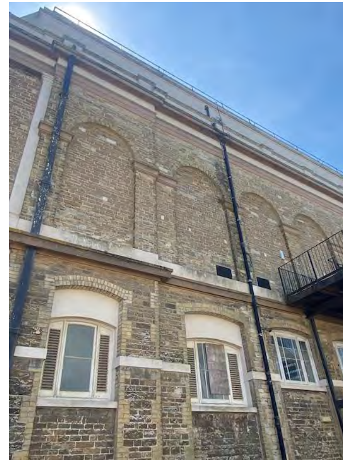
Louvered windows on the north elevation
