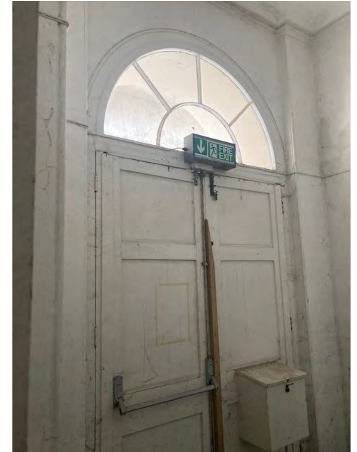
Main Entrance Doors
