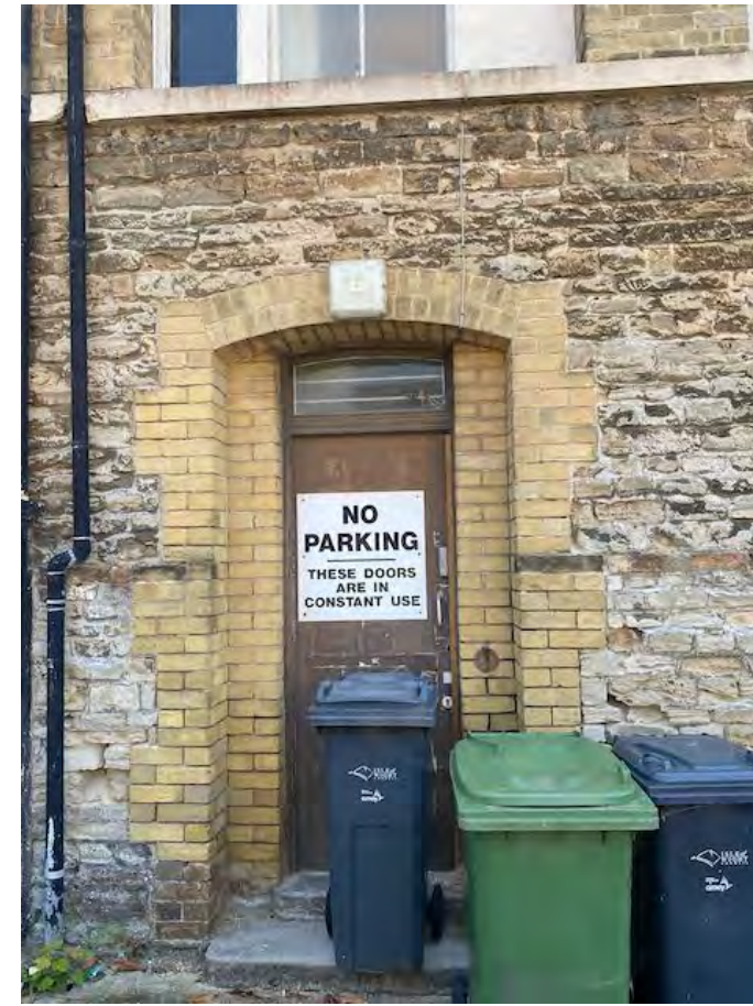
Downpipe on the northern elevation.
