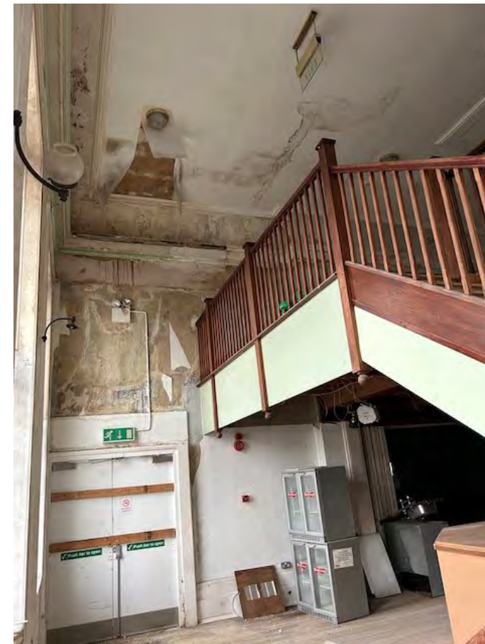
New mezzanine altering proportions of the hall
