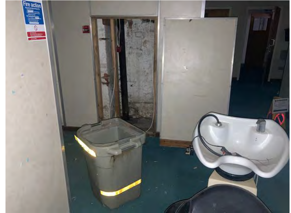
Area to the rear of the former entrance lobby
