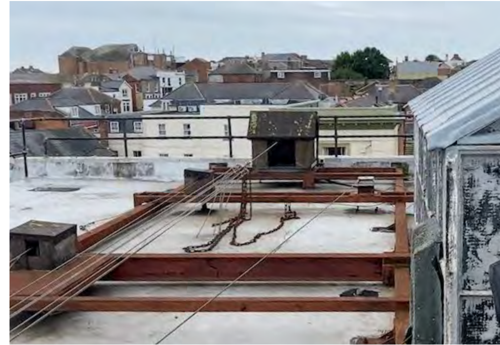
Steel frame structure for lifting scenery on the stage beneath
