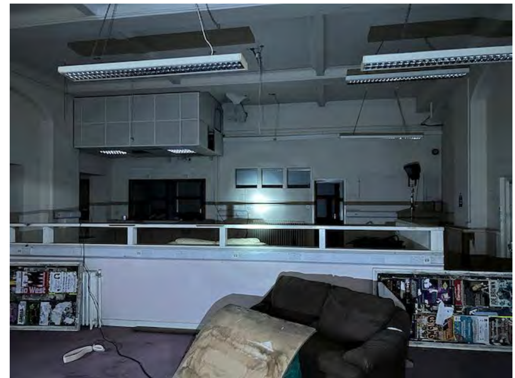
Lower main hall looking south
